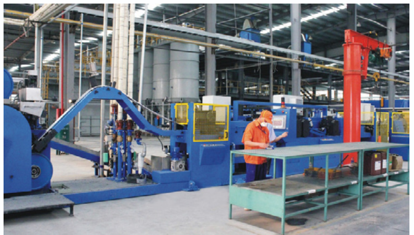
Strip casting production line
